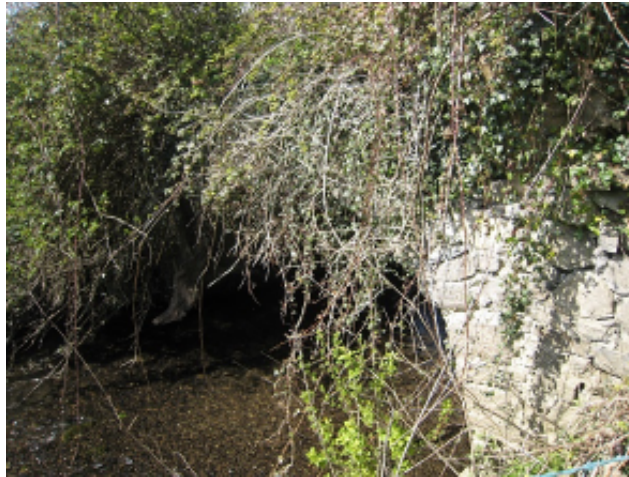
Plate 4: DU007-015007 Grace Dieu Bridge
